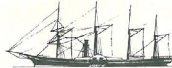
1838 GREAT WESTERN 1,340 tons First steamer built specially for the North Atlantic.
